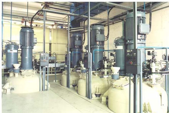
Top view of 4 High speed Turbo-mixers / dissolvers with capacity of 3.000 ltr. each
